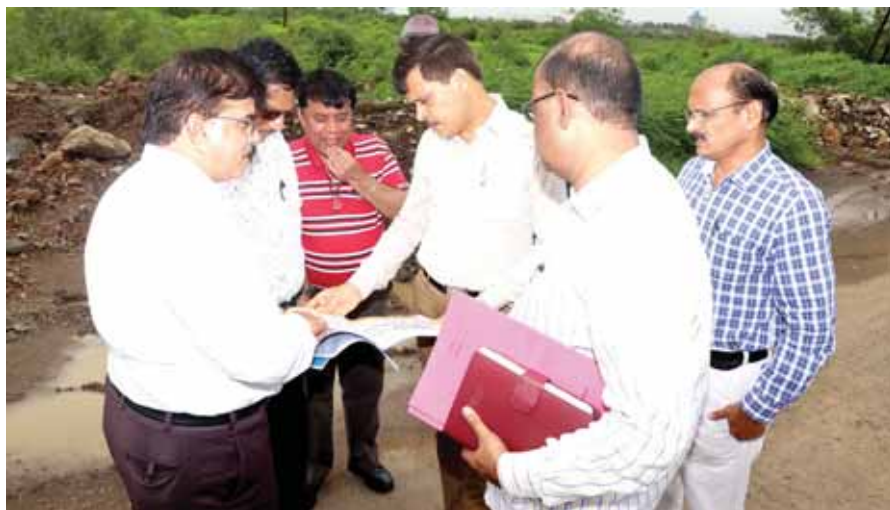
CIDCO's VC&MD Lokesh Chandra (3 rd from Right) reviews the developmental work at NMIA & Moha Creek sites.
